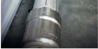
In Lewiston, Idaho, Mike's Mechanical installed MegaPress Stainless fittings in a high-tech facility manufacturing circuit boards for a broad range of products. During production, the boards are cleaned using high heat and corrosive chemicals, so the use of stainless steel pipe and fittings was essential.
