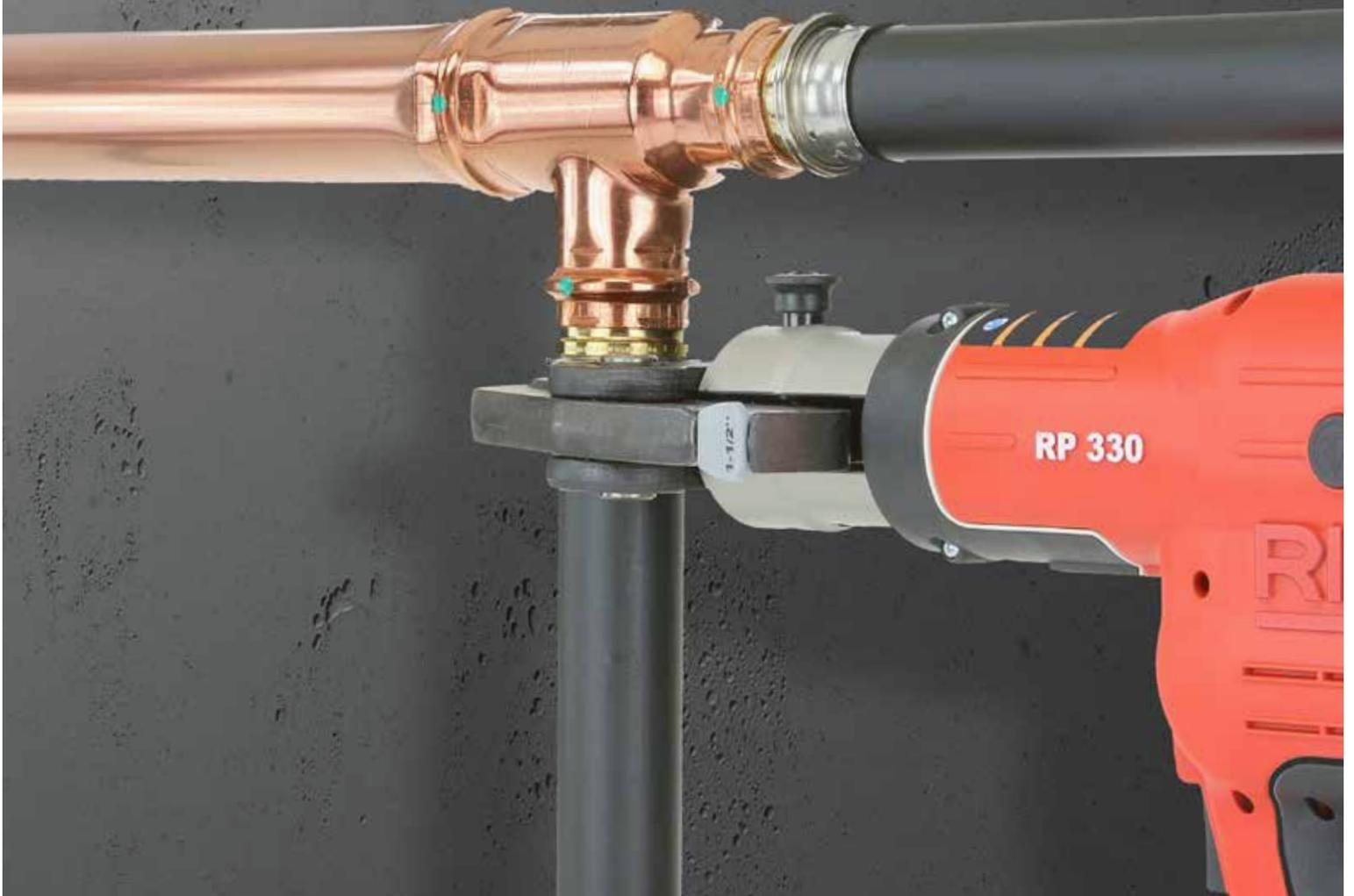
Trust Viega PureFlow System for your next commercial PEX installation. Choose a system that is free of solder, glue and the risk of micro tears in cold expansion. Viega's system allows for immediate pressure testing with connections made in seconds instead of minutes. Plus, the PureFlow tool platform is the only one in the industry that can be used for copper, stainless and carbon steel installations.
