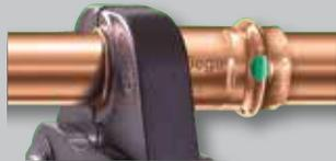
**2** Use the press tool to press the fitting, making a connection.
