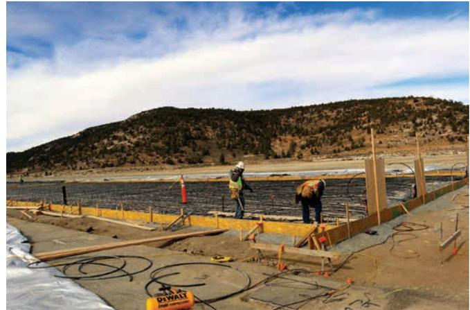
Since the facility produces its own electricity using three natural gas generators, the water flowing through the slab would be heated with a heat exchanger in one of the generator’s exhaust, making it an efficient co-generation system. Within the first year alone, the new system has saved approximately \$200,000 in transportation and fuel costs.
