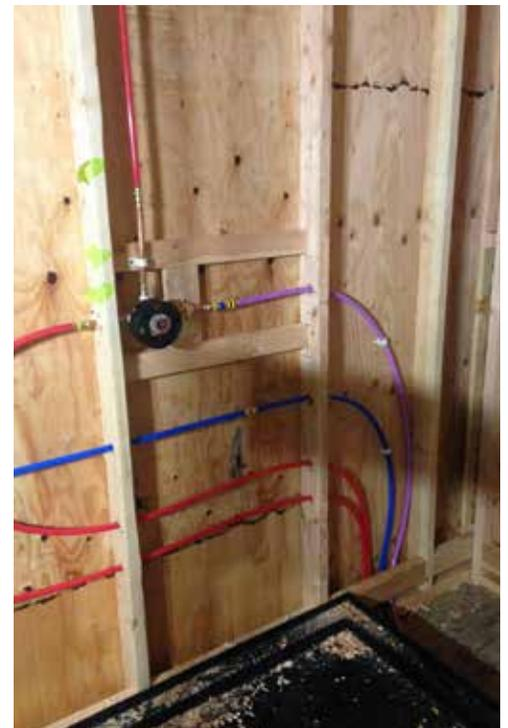
Viega PureFlow System was used to circulate hot and cold potable water in the tiny house, as well as reclaimed water.
